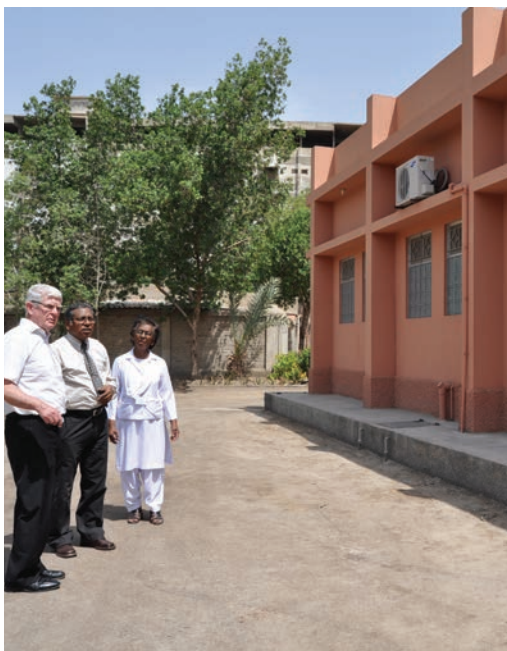
Newly constructed diagnostic laboratory.
